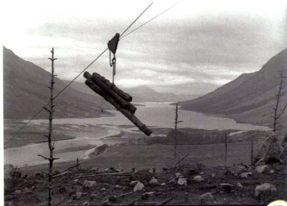
Blondin tackle wire ropeway being used by Canadians on Loch Etive, 1944
