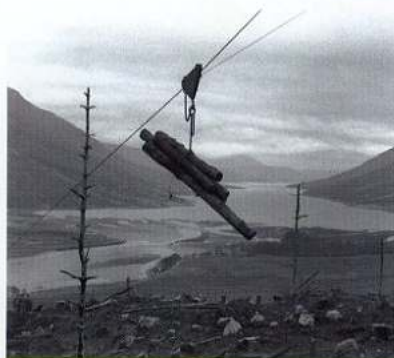
Blondin tackle wire ropeway being used by Canadians on Loch Etive, 1944
