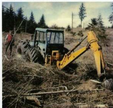
Backacter digger in action, draining recently felled wood, 1979
