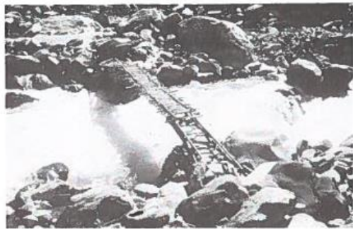
● Timber bridge over a raging torrent.
