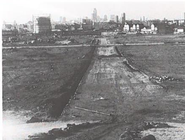
● Looking towards the London skyline from development. The two photographs, taken at different times, show the dramatic transformation of the site from No
