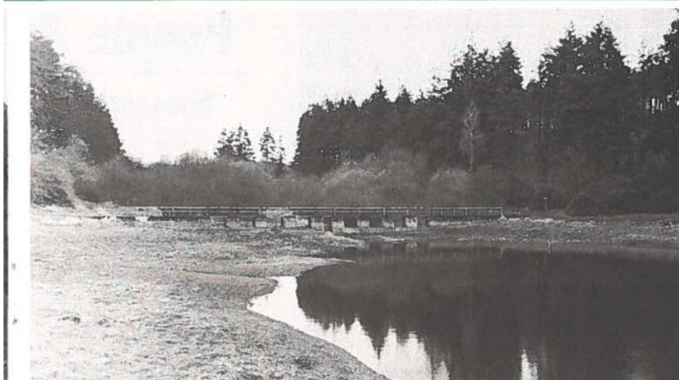
● The sluice above Trenchford Reservoir.
