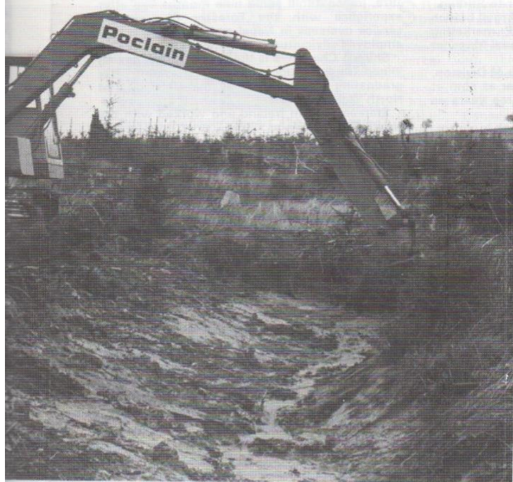
● Restoring the drainage system.
