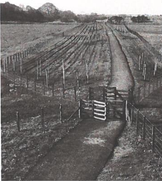
• Tree planting, fencing and footpath construction for Irvine Development Corporation.
