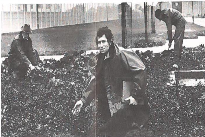
Douglas Lamont supervises shrub bed work at HM Wayland Prison.
