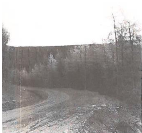
he formation of a new forest road through the plantations of Ben Newe. Extraction racks from a previous thinning in the pine can be seen in the background.
