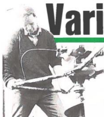
Squad foreman Alex Henderson augers post holes for a screen fence at Brickfield, Craigellachie, for main contractor Robertsons of Elgin Limited.
