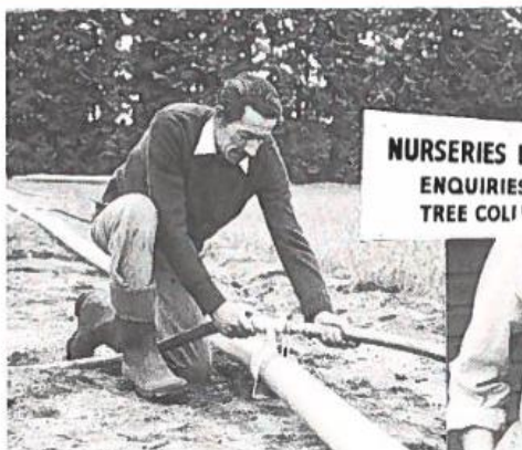
● Charlie Scott assembling irrigation pipes.
