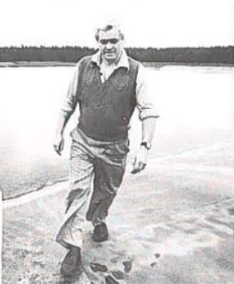
● John Simmons makes a routine inspection of one of the reservoir liners for possible damage.
