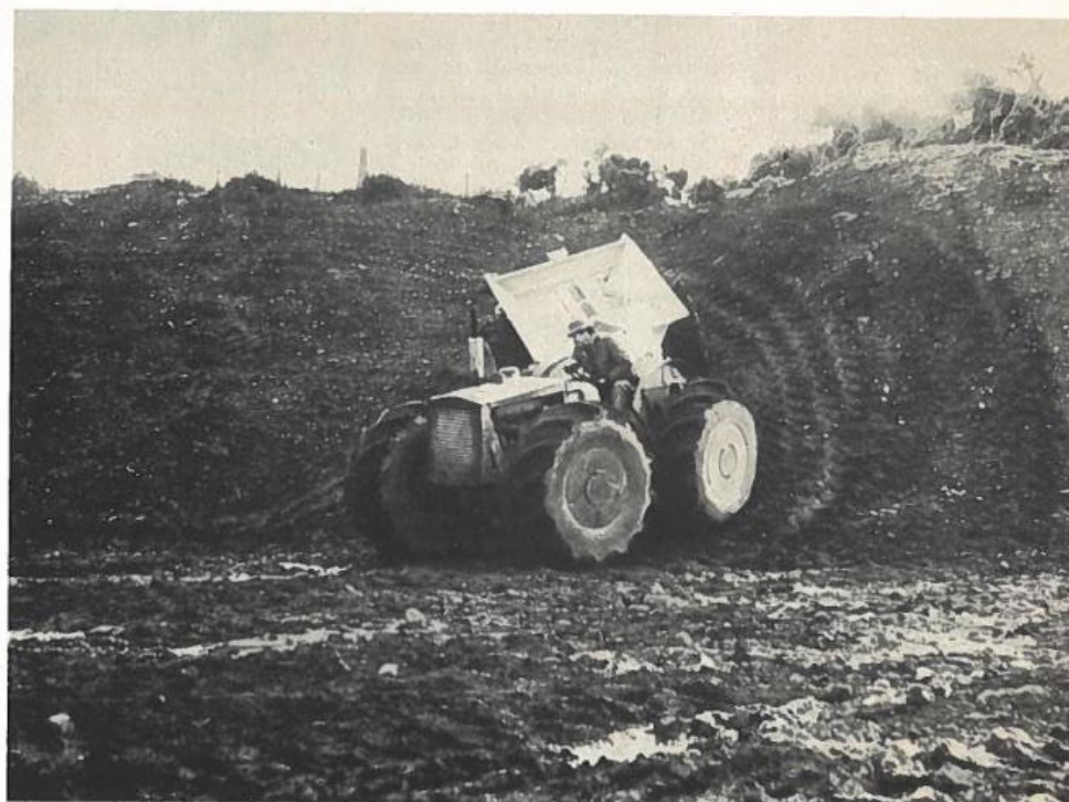
The preparation and seeding of 3.65 ha was part of a land improvement scheme at Brora in Sutherland, funded by the SDA. The area constituted the slopes of the large arena and surrounding a proposed games pitch; built on the site of the old Brora brickworks and coal mine.
