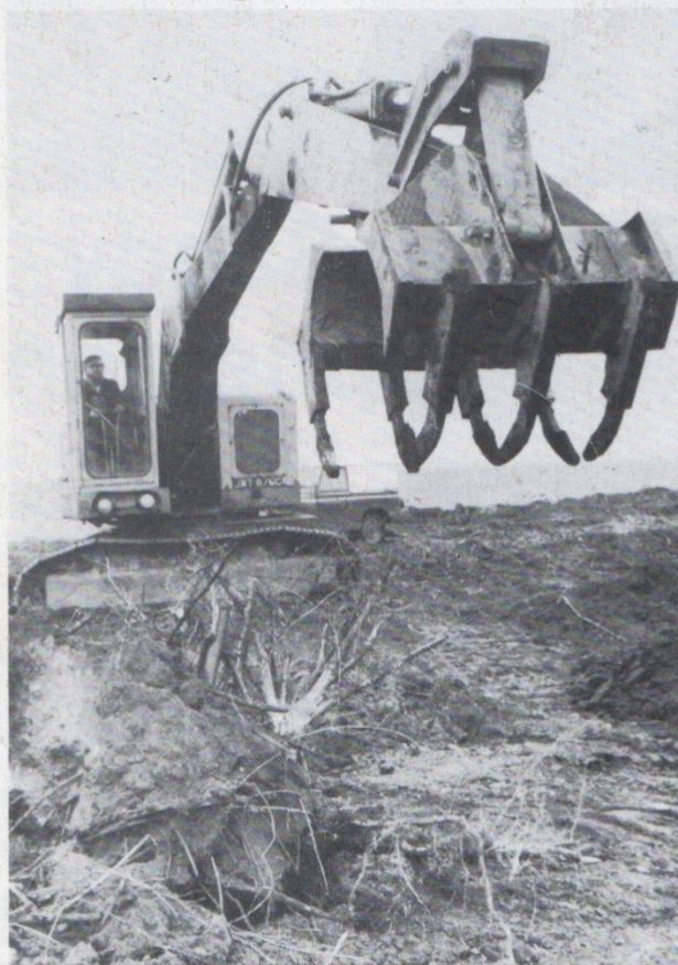
Purpose-built mechanical grab at work in East Anglia —see Better Land Use on pages four and five.
