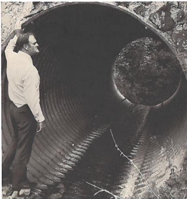
Top: Crossing a gully or 'sike' — Peter Sloan shows the scale of a forester's rudimentary but practical bridge formed by placing a large diameter culvert pipe, and infilling.
