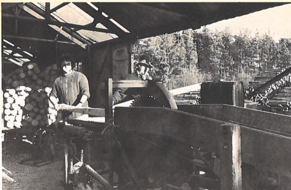
After the stake lengths have been peeled and graded, they are pointed as shown here and banded into pre-determined bundle size, before going for air seasoning.
