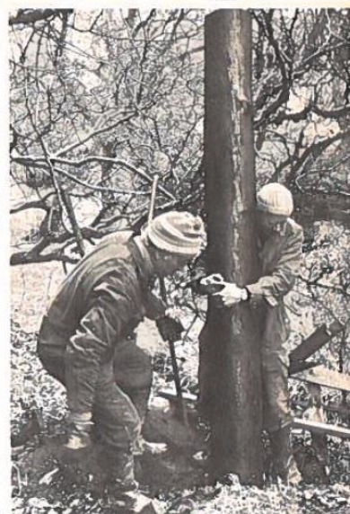
Jeffrey Graham and Ian Thomson manhandle a straining post into position. . . . .
