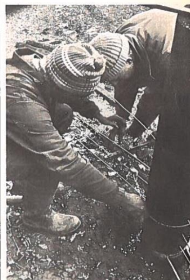
. . . . . and tension the wires of the new fence.
