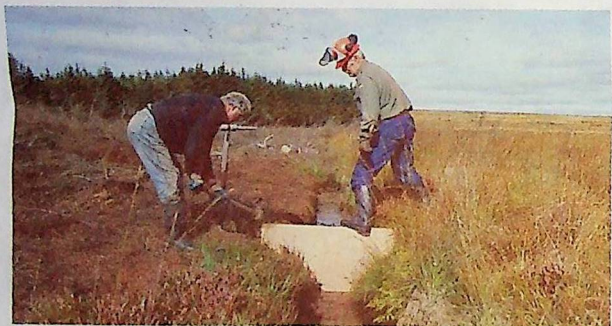
● Work already under way . . . blocking drains on the mire sites.
