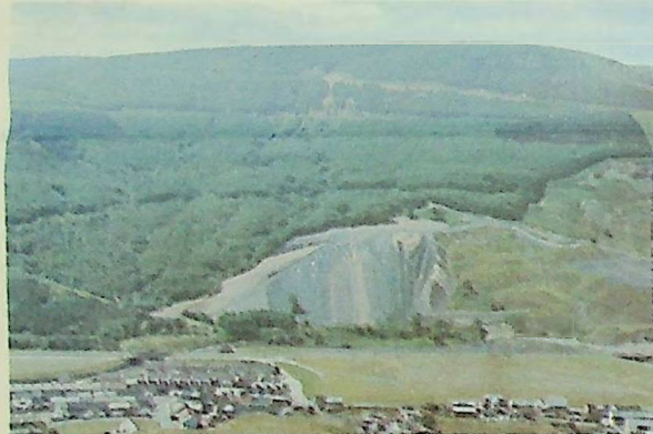
View visitors had of Lady Margaret Tip now being re-shaped by Commission. This will be eventually planted.
