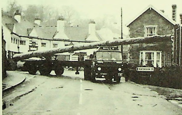
The pole being manoeuvred through Tintern Village.
