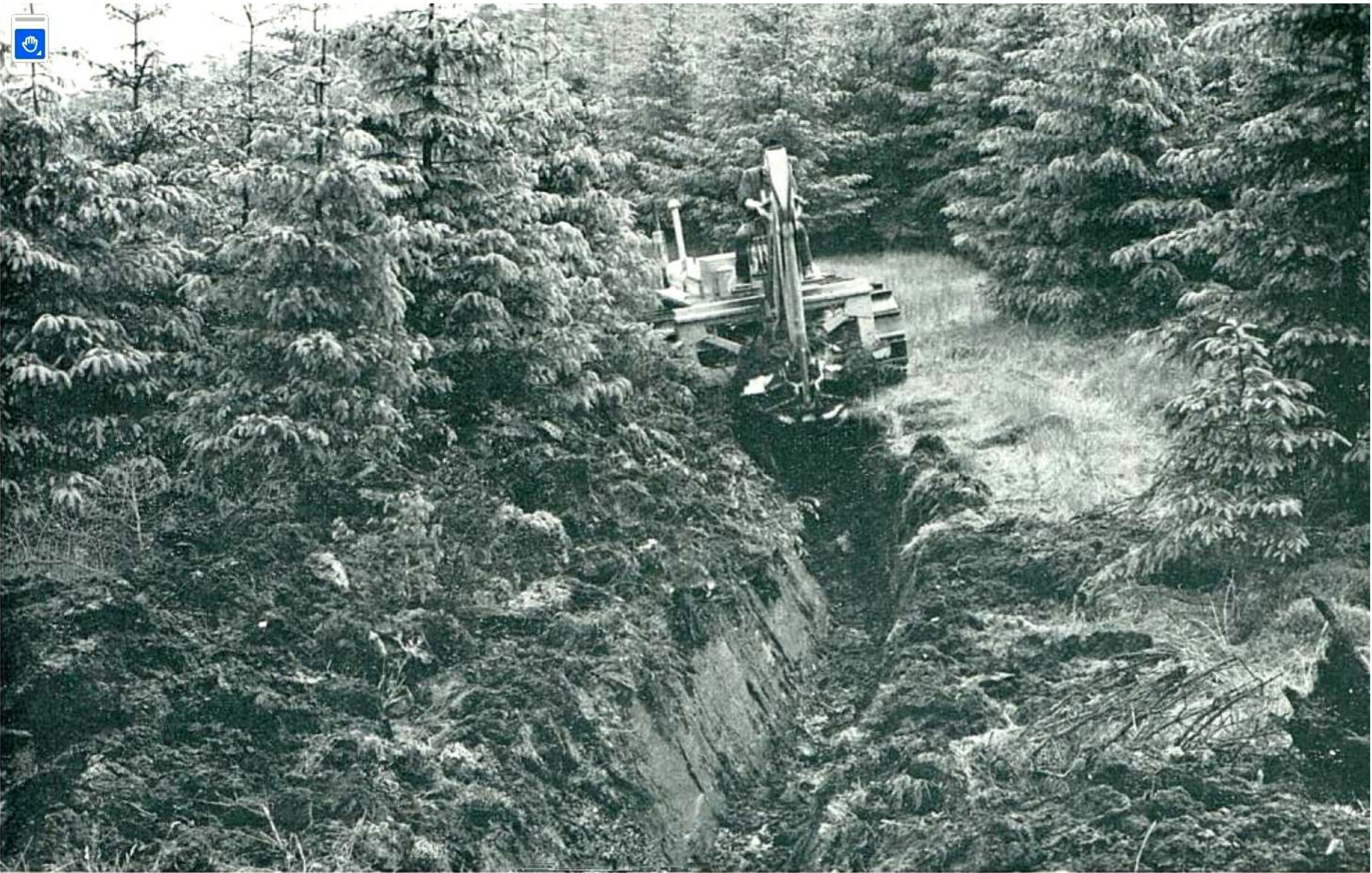
PLATE 6. Digging a deep drain in Carron Valley Forest, Stirlingshire, using a back-actor excavator powered by a crawler tractor. Deep drainage of this heavy clay soil is designed to bring spruce plantations out of "check", and raise their Production Class.
