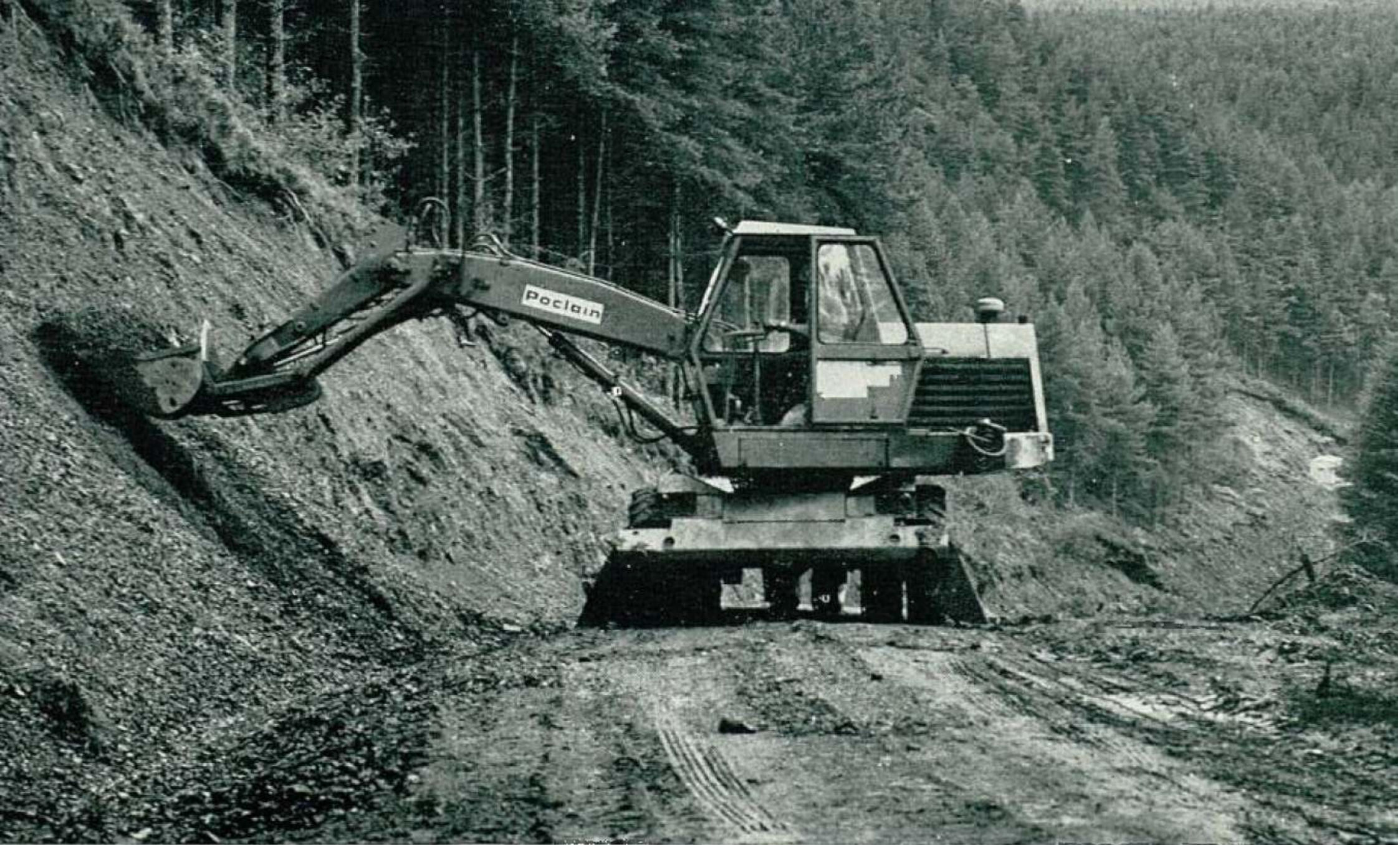
PLATE 15. Road construction. A giant powered shovel excavates a road bed formation out of a steep hillside at Rheola, in South Wales.
