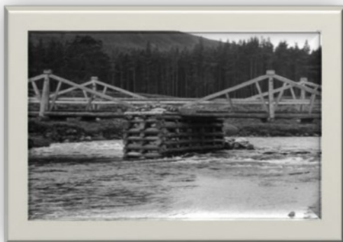
This timber bridge over the River Dee has all the hallmarks of the Canadian Forestry Corps. Timber products were taken for onward transport by light rail. Forestry Memories website. [Beautifully constructed! -Ed]
