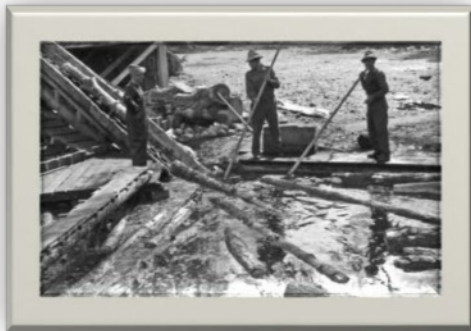
CFC co. no 25, Mar Lodge camp logging pond. Ponding removed mud and stones from logs, reduced saw damage and allowed logs to be sorted. Forestry Memories website. [Some of those logs look fairly dodgy quality! -Ed]
