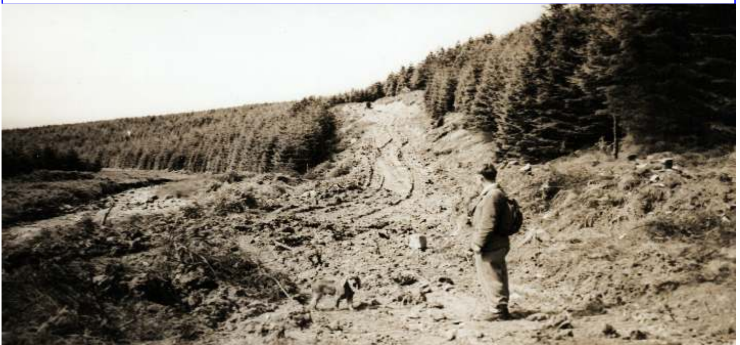
Construction of the first forest road in Newcastleton Forest to the Kershope Burn (and thus to the Kershope Forest and England), August 1950. The author is in the foreground.
