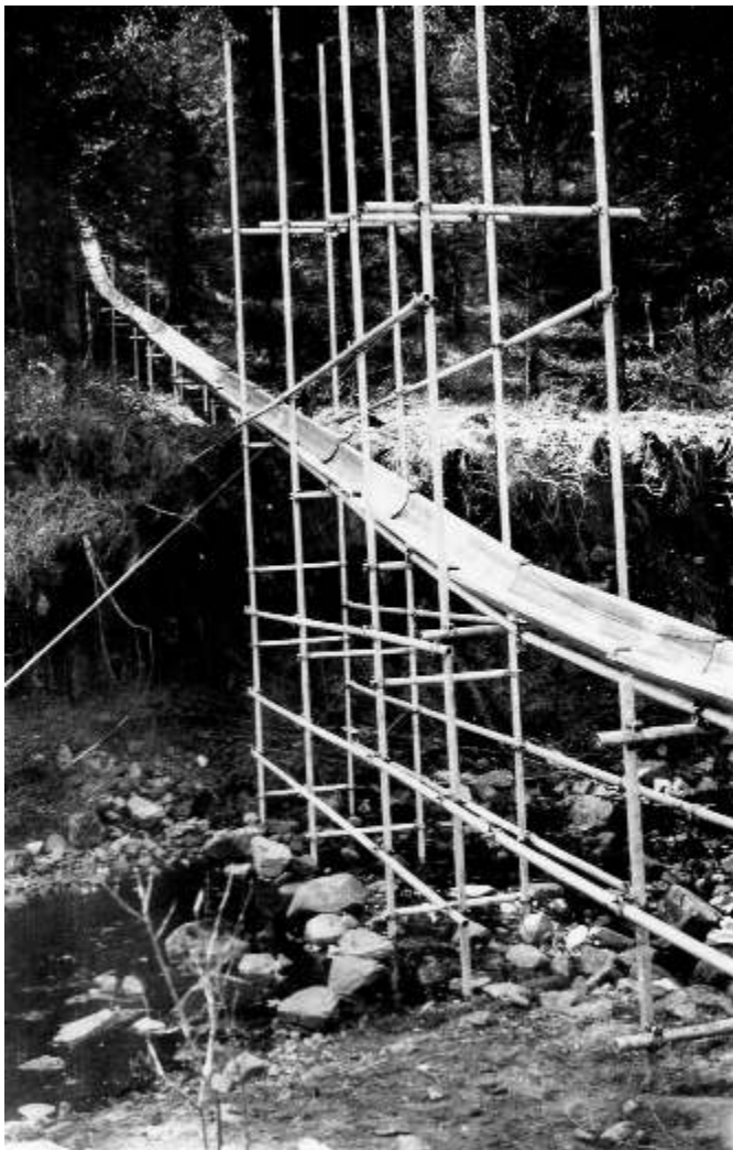
Aluminium chute crossing the Tweedenburn on tubular scaffolding. Newcastleton, May 1951.
