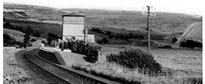
Plashetts Colliery incline is on the right
