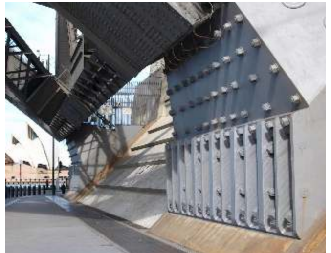
The Bridge has six million rivets
