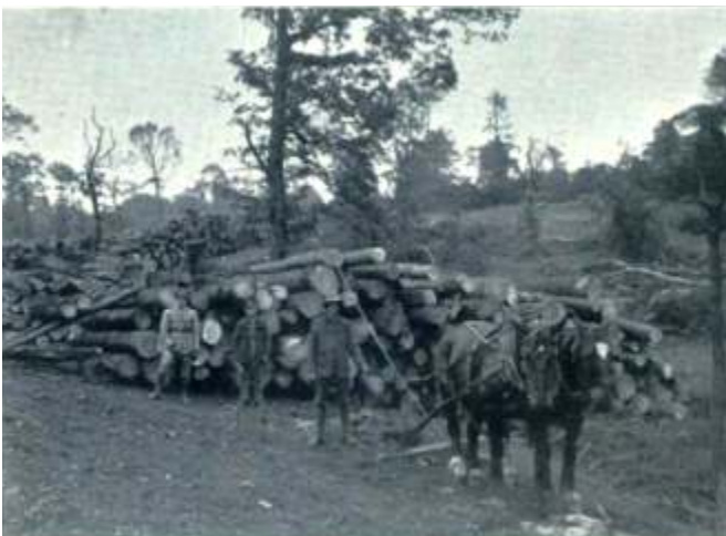
Piling logs in Scotland
