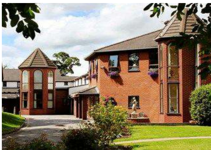
Beaufort Park Hotel in Mold
