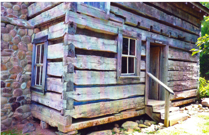
The settlers in the 19 th & 20 th centuries built everything out of wood - except the chimney!
