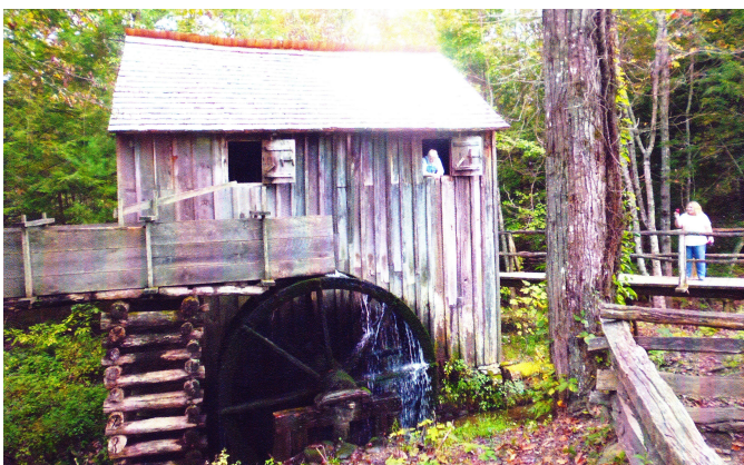
The working watermill - everything but the millstones from wood.
