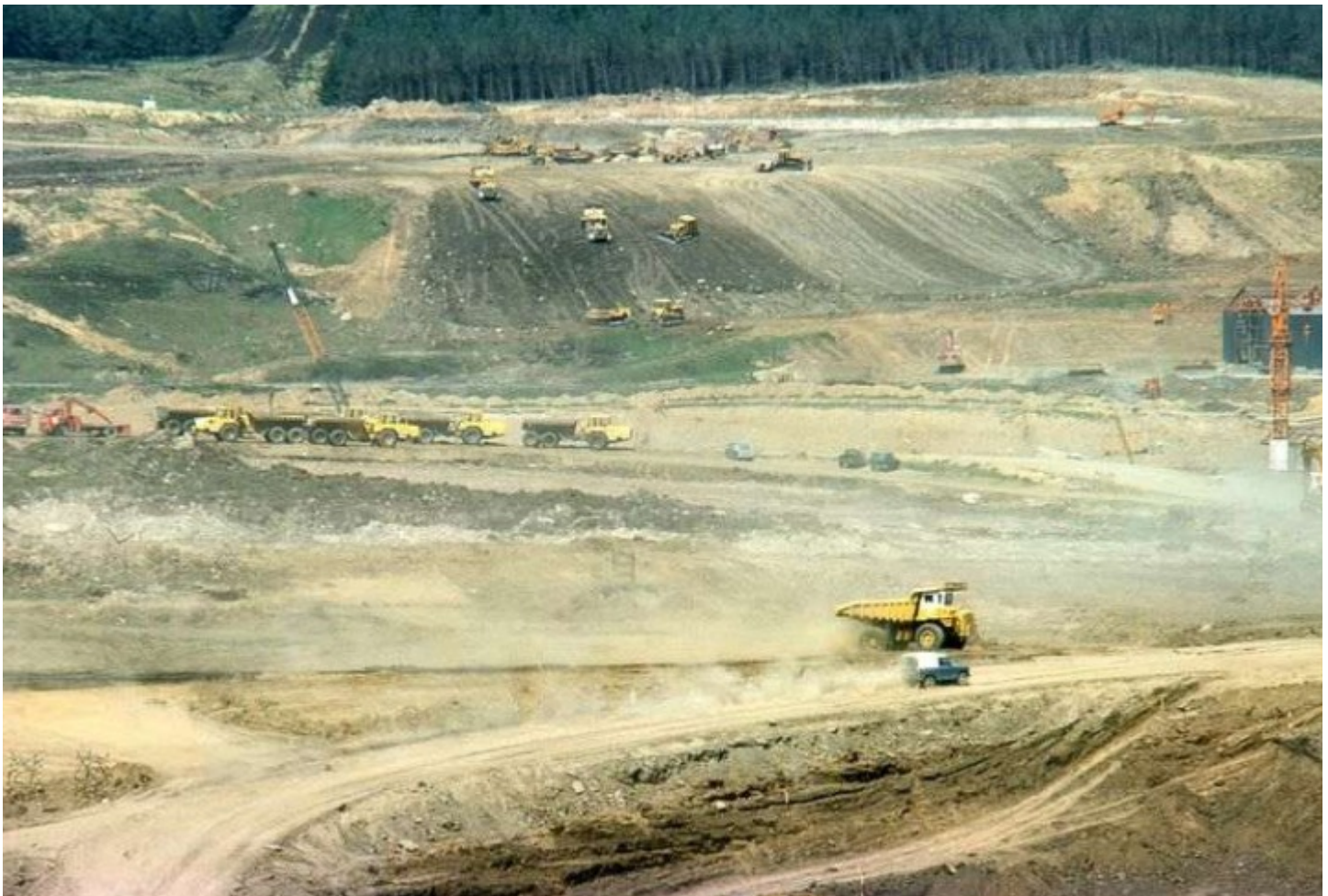
Kielder reservoir under construction in 1972
