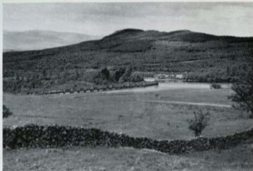
Dundeugh Forest and a Hydro-Electric Dam
