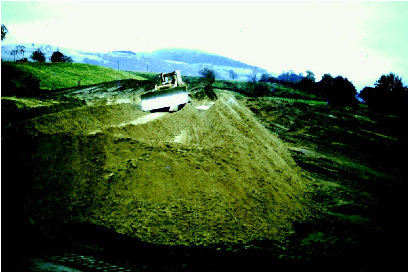
This photograph shows a bulldozer working a gravel deposit on the neighbouring farmland at Duireaskin in order to form the entrance from the A827, together with the section of forest road from the A827 up to Burnside.
