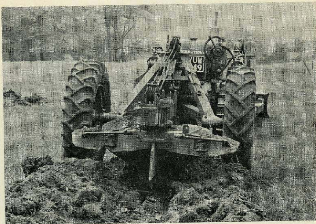
Pl. 17. An early version of the double mouldboard tine plough mounted on a "Universal Carriage." (Forestry Commission A2285).
