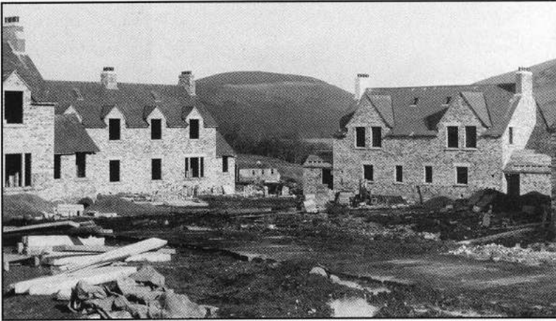
Constructing the first houses of Ae village
