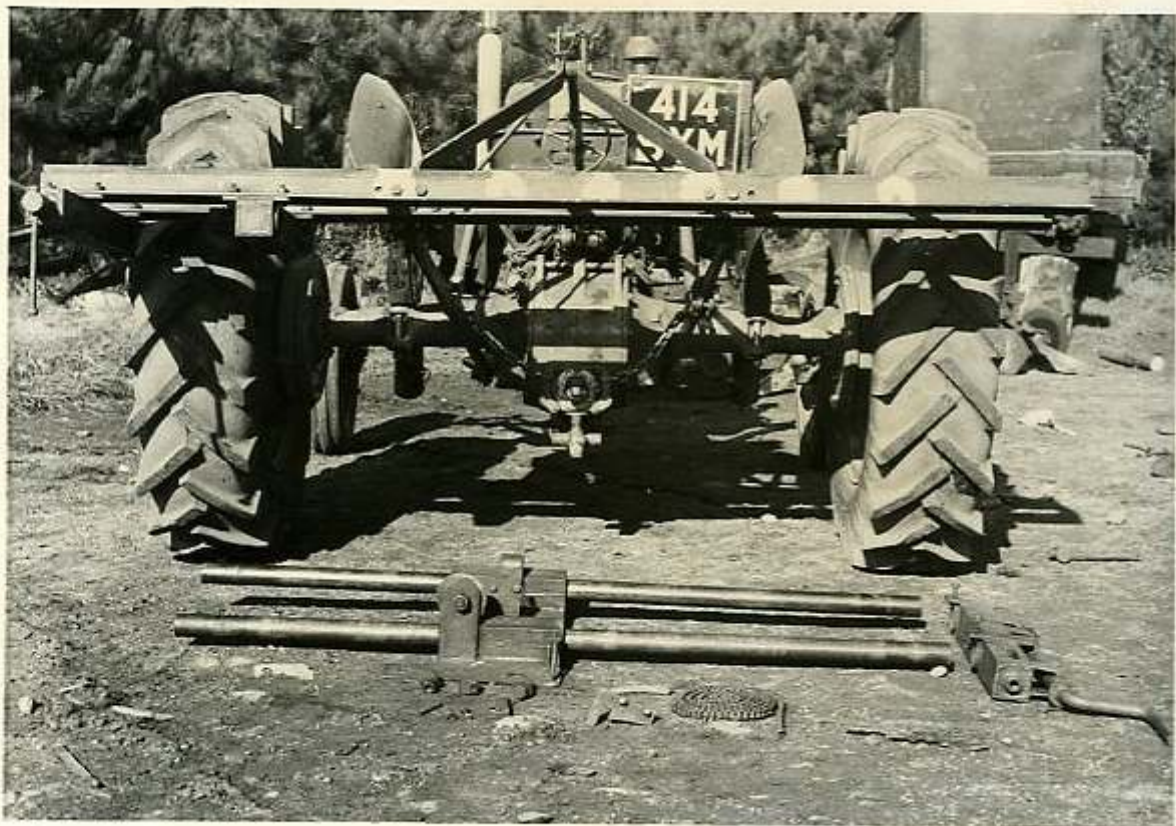
Tool Bar Frame on 3 Point Linkage
