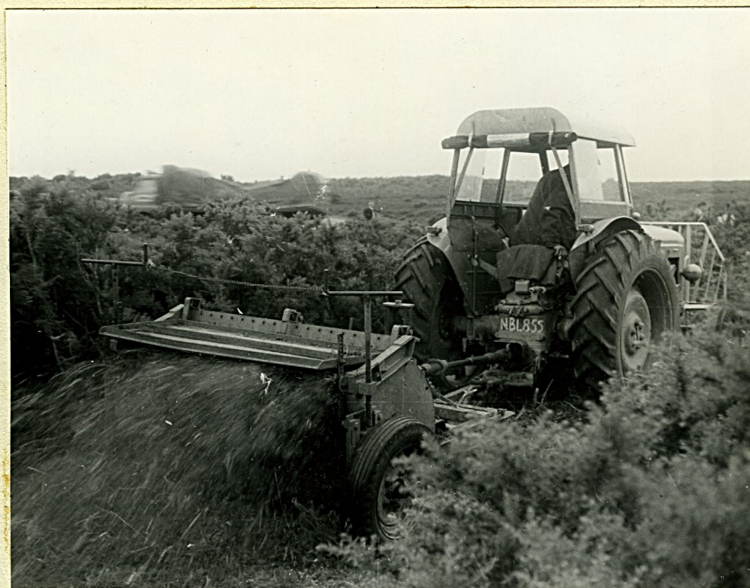
5. The Wilder Rainthorpe cutting gorse. Note the finely shredded debris coming out of the back of the machine.
