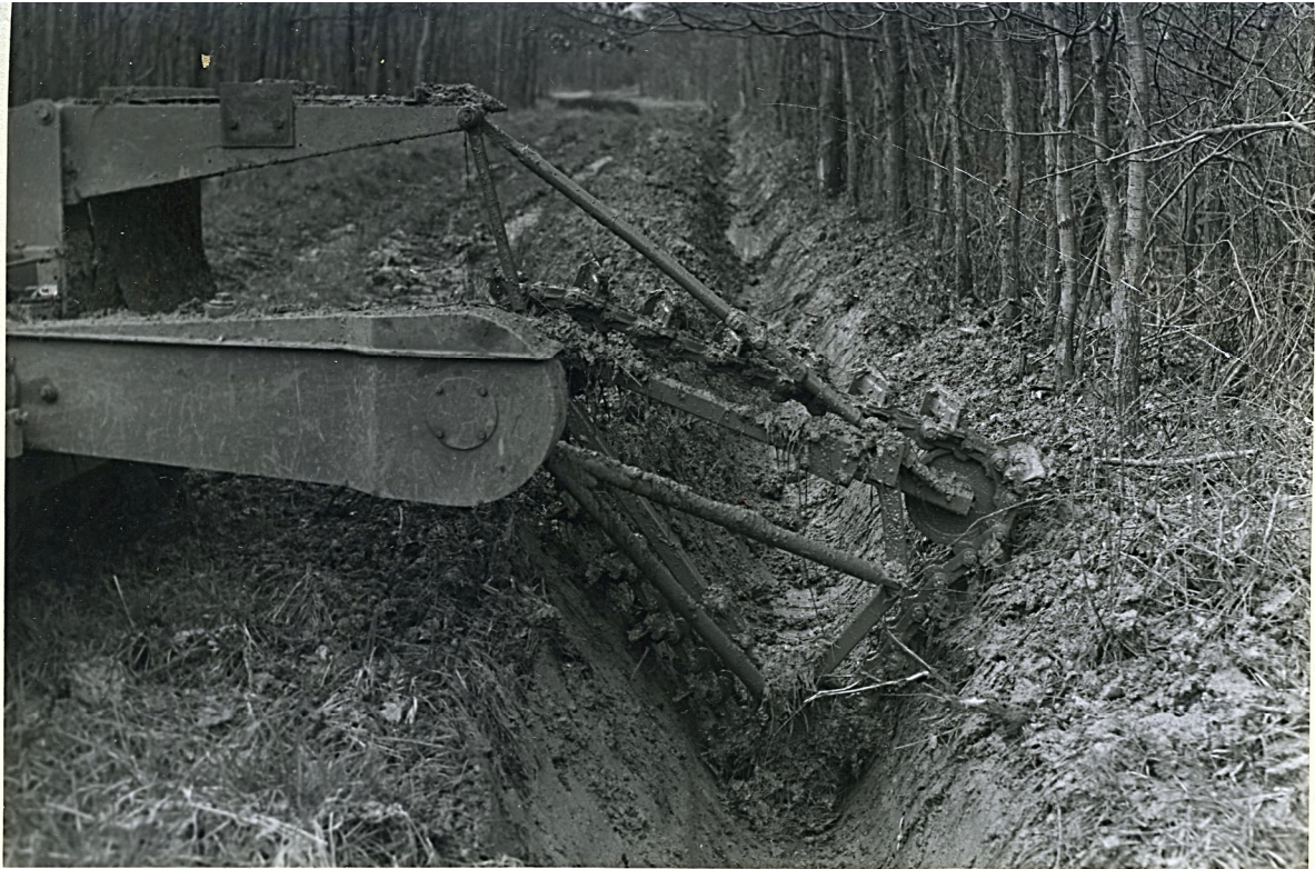
Photograph 1. The machine is here seen doing a third cut to complete the restoration of a drain in a clay soil.
