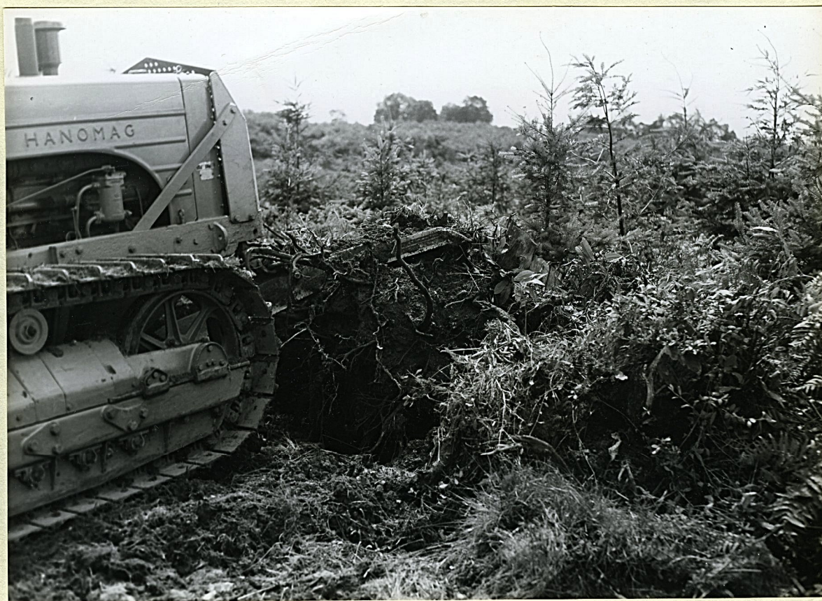
Photograph 3. The two large coppicing Chestnut stumps referred to at Observation 4. Note how the stumper has worked round the front and sides of the stumps without damaging the standing crop behind.
