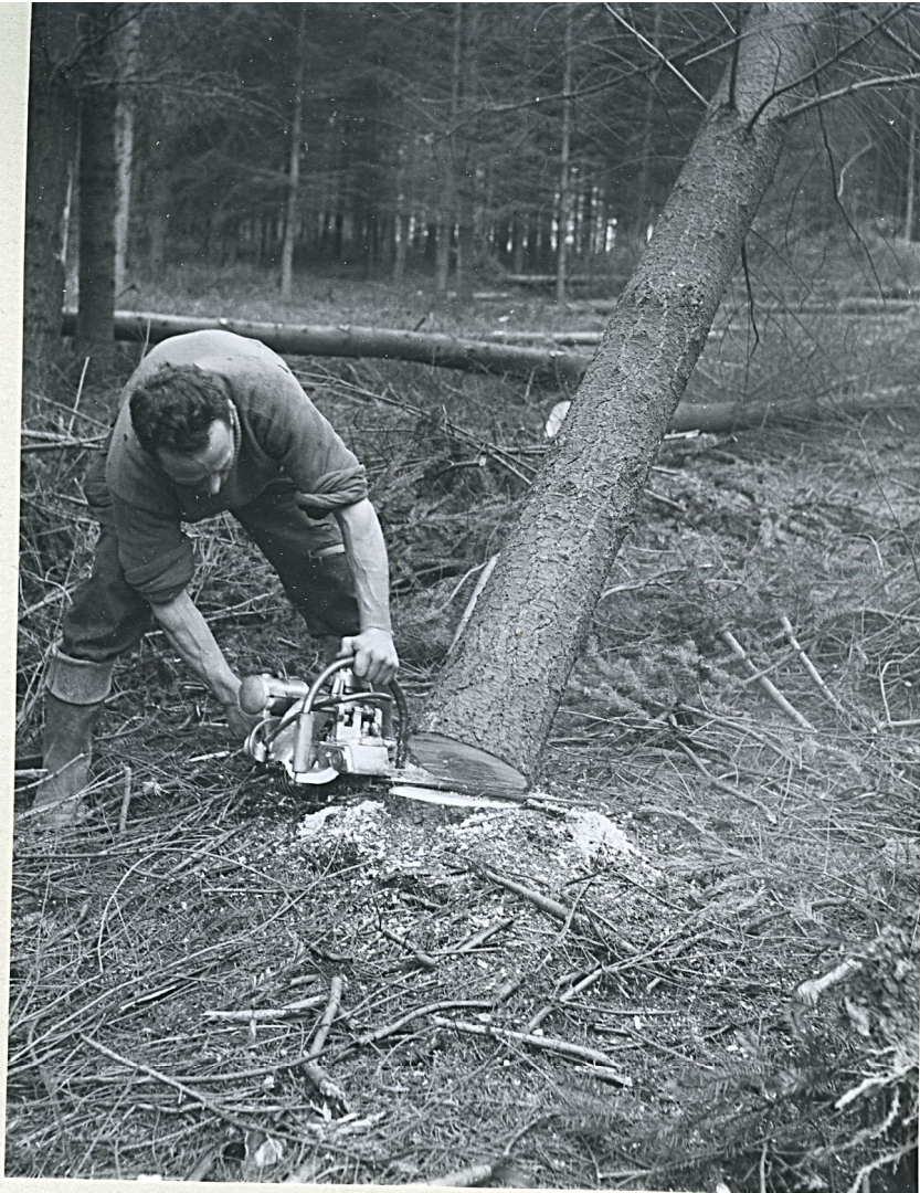
PHOTOGRAPH 3. - Felling (note the low stump).
