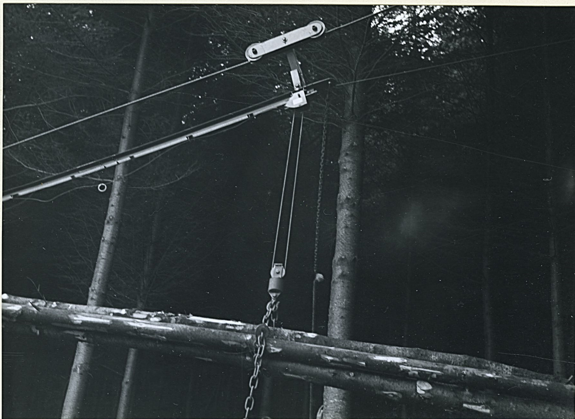
PHOTOGRAPH 2. Showing the load being raised to the carriage.
