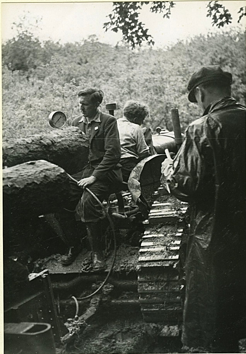
THE METHOD OF INSERTING THE DYNAMOMETER FOR RECORDING ROLLING RESISTANCE
