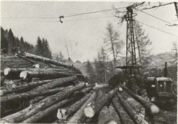
Back in the UK an Alp owned by EFG in Ardgarton demonstrates how a skilful operator can turn logs on arrival at the roadside. This gives more landing space for log storage and allows loading out without stopping the winch.
